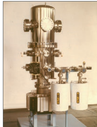
1973 Ultra-high vacuum evaporation with metal bell housing.
